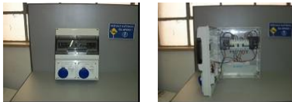
Figure 4: Front and internal views of recharge panels for cars
